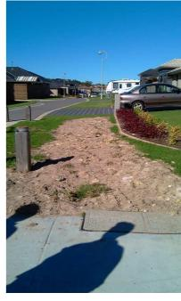
This is a carriageway and shoulder failure as a result of excess vehicles due to M2M project. The carriage way has been made safe and it will be repaired once M2M has been completed.
